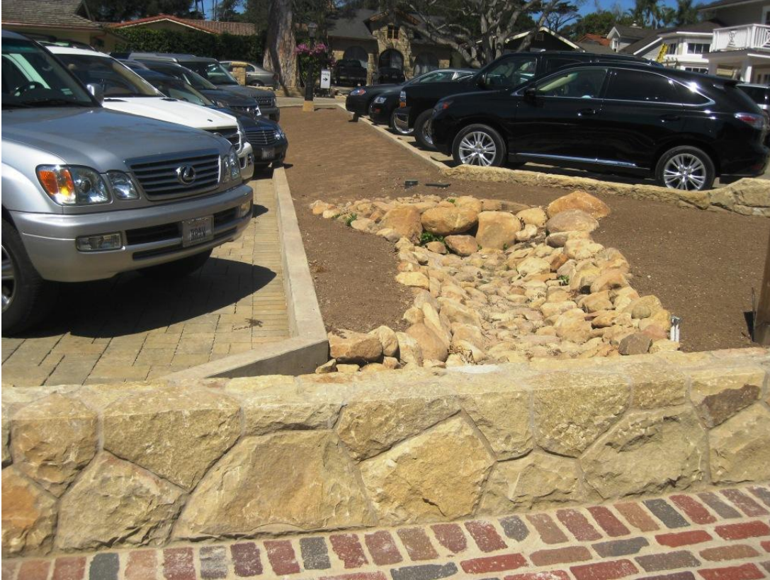
Gunner Commercial Redevelopment, San Ysidro at E. Valley Road in Montecito
