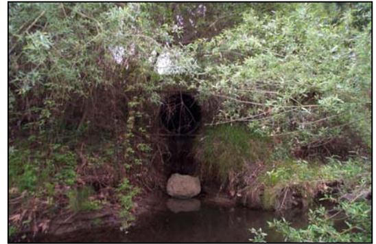
Storm drain inlet to Arroyo Burro (AB-2)
