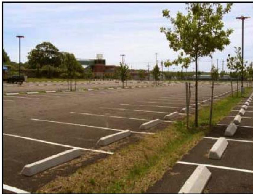
Figure 5 – Porous Asphalt Parking Lot, University of Rhode Island, Kingston (Source: [http://efc.muskie.usm.maine.edu/docs/LID\\_Fact\\_Sheet.pdf](http://efc.muskie.usm.maine.edu/docs/LID_Fact_Sheet.pdf))
