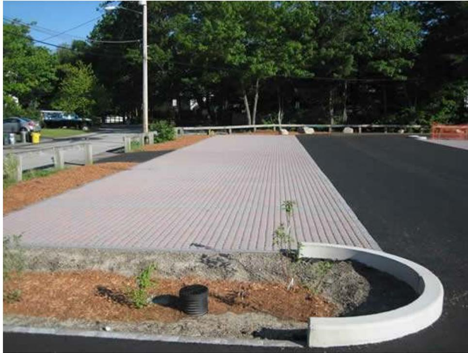
Figure 4 – Permeable pavers, porous asphalt, and bioretention cells at the Silver Lake beach parking lot, Wilmington (Source: GeoSyntec Consultants)
