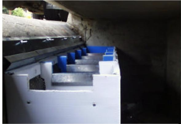
*Stormwater filter installed in a catch basin in Goleta as part of a pilot program*
